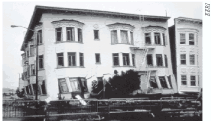
Figure 68 - Liquefaction caused differential settlement under this building and increased damage during the Loma Prieta Earthquake.
