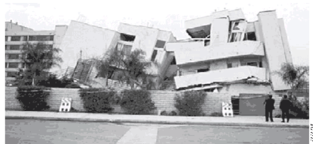
Figure 32 —This modern wood-frame apartment building had a central driveway. It collapsed inward over unbraced entrances to crush first-story parking during the 1994 Northridge earthquake.
