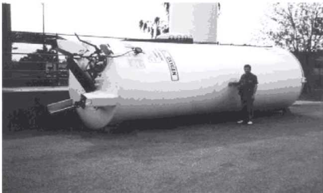
Figure 46 - The support pedestal system of this oxygen tank at Olive View Medical Center was damaged after the 1994 Northridge earthquake, leaving the tank leaning. The tank is shown after it was removed to allow for installation of a replacement unit.
