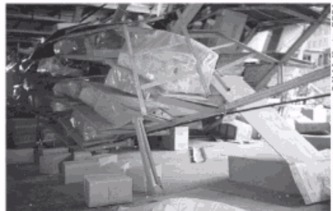
Figure 42 - The storage rack collapsed in this warehouse-style retail store during the 1994 Northridge earthquake. Heavy items such as the sofa in the center of the photo crashed to the ground and could have injured employees and shoppers.
