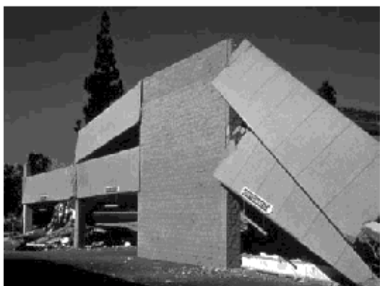
Figure 5 - Concrete Parking Structure Collapse.
