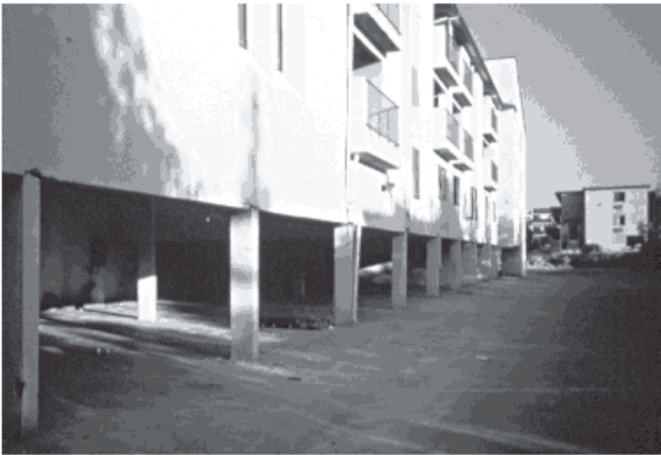
Figure 30 —Apartments with tuck-under parking like this can collapse. This building is leaning but did not collapse in the 1994 Northridge earthquake.
