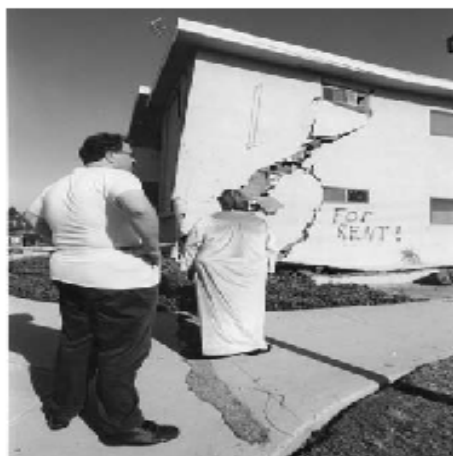
Figure 2 - Northridge Earthquake, Jan 17, 1994. Collapse of the lower, soft story of this apartment rendered it uninhabitable.
