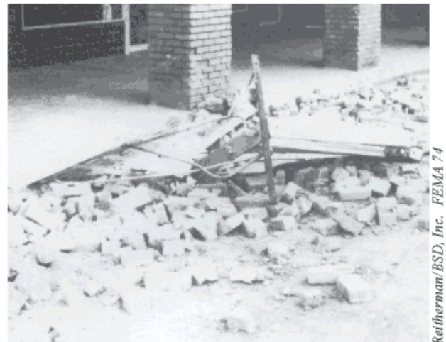
Figure 38 - The sign on this commercial building fell in the 1979 Imperial Earthquake.
