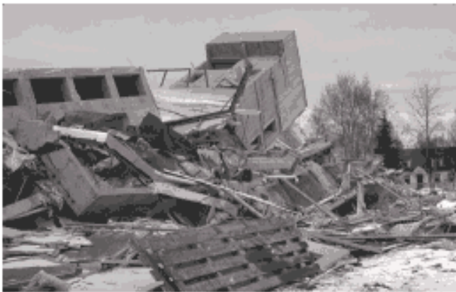
Figure 33 - This six story lift slab building collapsed in the 1964 Alaskan Earthquake.
