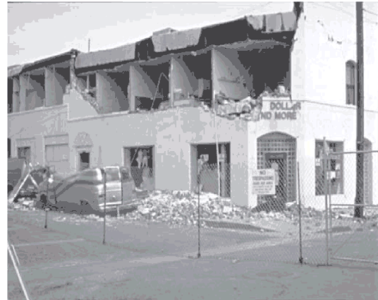
Figure 16 - The second-story wall of this unreinforced masonry building was not well-tied to the roof, and the building collapsed during the 1994 Northridge earthquake.
