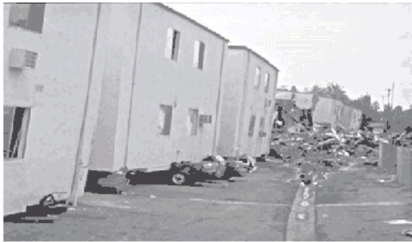
Figure 31 —A similar apartment building's soft story collapsed on cars during the same earthquake.
