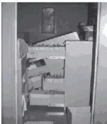
Figure 3 - File cabinet drawers can slide open and unbolting cabinets can topple during earthquakes.
