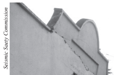
Figure 18 - Parapets. They are the tops of walls above the roof can fall off buildings like this one nearly did in Rio Dell during the 1992 Cape Mendocino Earthquake.
