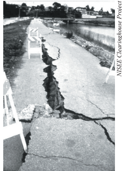
Figure 67 - Lateral Spreading. Loma Prieta Earthquake, October 17, 1989. Lateral spreading damage levee road along the San Lorenzo River.
