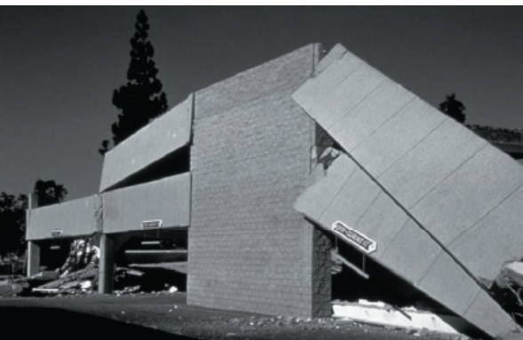
Figure 5 - Concrete Parking Structure Collapse.
