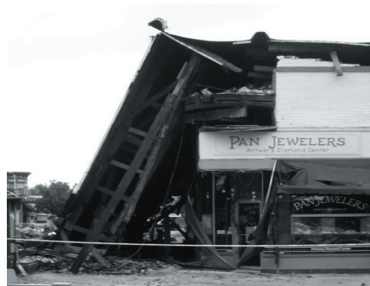
Figure 6 - San Simeon Earthquake, Dec. 22, 2003. The Acorn Clock Tower Building constructed of unreinforced masonry collapsed killing two people.
